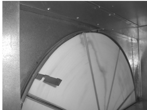
Figure 10. Pull the segment up and out of the wheel frame to remove
