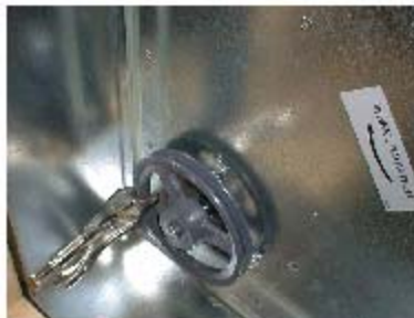
Figure 13. Secure pulley and belt with vise grip to prevent wheel rotation.
