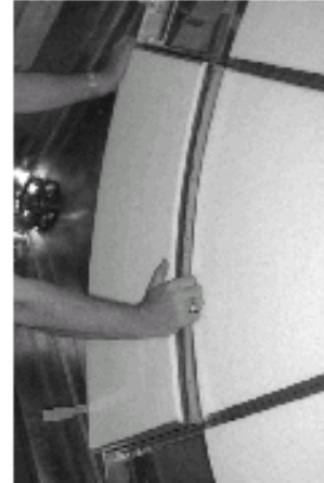
Figure 15. Install outer segment by starting lower end in position and pressing straight in
