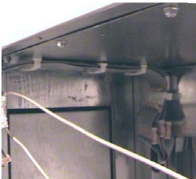
Figure 6. Energy wheel modules may have factory-installed ribbon cables attached inside. Take care when penetrating the unit casing.
